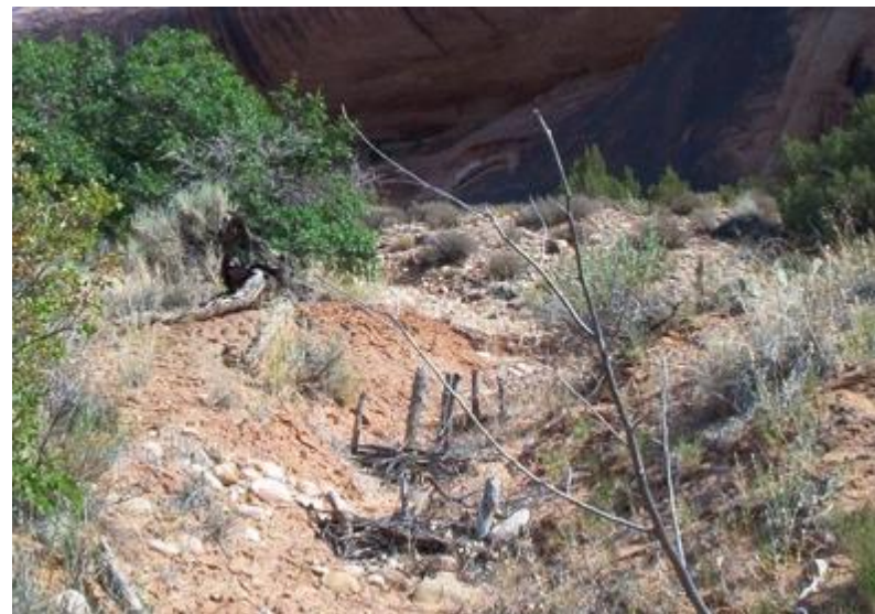
Figure 8: Example of erosion control with wattles and brush fences. Photo: K. Dohrenwend 2003
